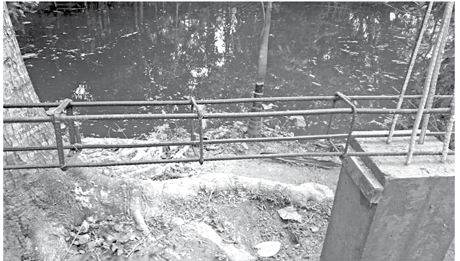
Rebar rings are being used around 15 inches apart from each other in a lintel for the under construction boundary wall of Babur Bazar Government Primary School in Moulvibazar's Rajnagar upazila.
