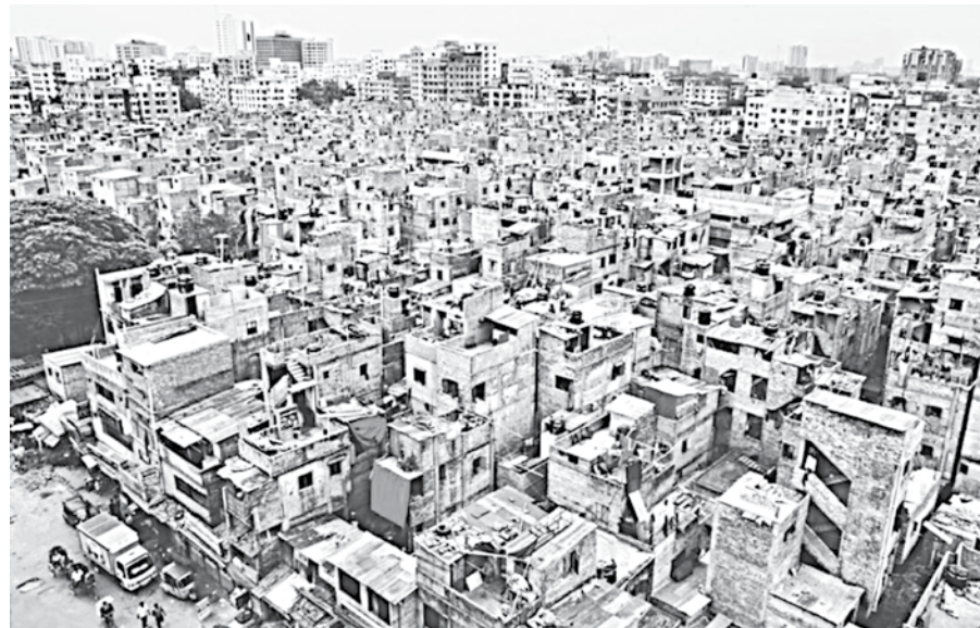
A major earthquake may cause massive destruction in the highly populated capital crammed with unplanned buildings, like that seen in this picture from Mohammadpur.
