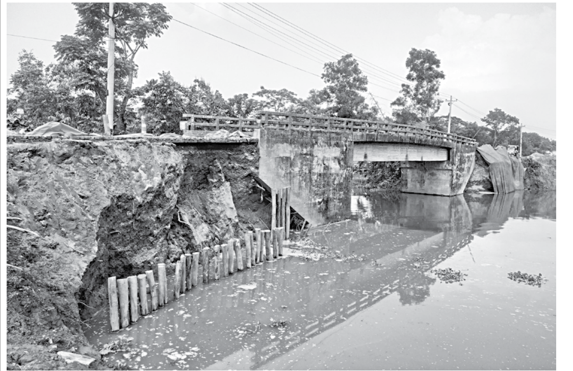
Roads and Highways Department in Kishoreganj recently placed wood logs to stop further erosion of an approach road to this bridge on Bogaputa canal in Ishwarganj upazila of Mymensingh. PHOTO: COLLECTED
