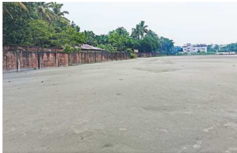
The partial view of an industrial estate of BSCIC in Kawnia, Barishal. The photo was taken yesterday.
