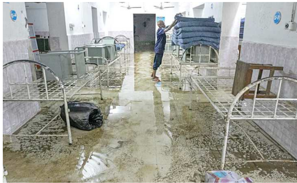
An employee of Ma O Shishu Hospital in Chattogram stacks the mattresses on a bed yesterday. The floor of the ward is filthy and wet as the ground floor of the healthcare facility had been inundated due to heavy rain in the port city the day before. The patients had to be moved to floors above.
