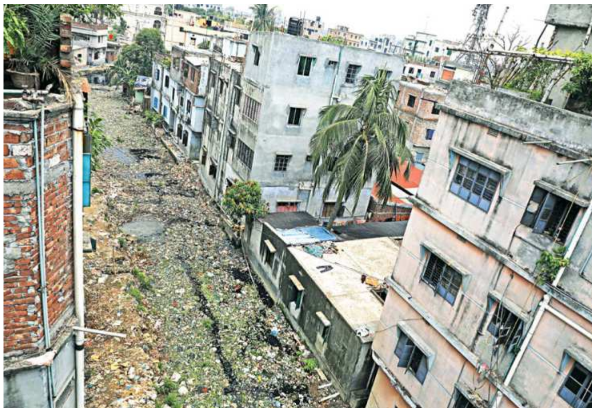
People discard bottles, containers, and polythene bags into the capital's Shyampur canal, polluting the water and clogging the canal. Water stagnates and the canal becomes a breeding ground for mosquitos. Its cleanup and development work has been halted for a long time. The photo was taken on Saturday. PHOTO: AMRAN HOSSAIN
