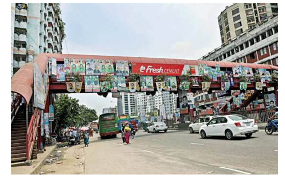
From the outside, little can be seen of this overpass at Kalyanpur Bus Stand area, as political posters have taken up almost all of it. It's worse from the inside, as pedestrians using it can see almost nothing going on outside. This photo was taken on Wednesday.
