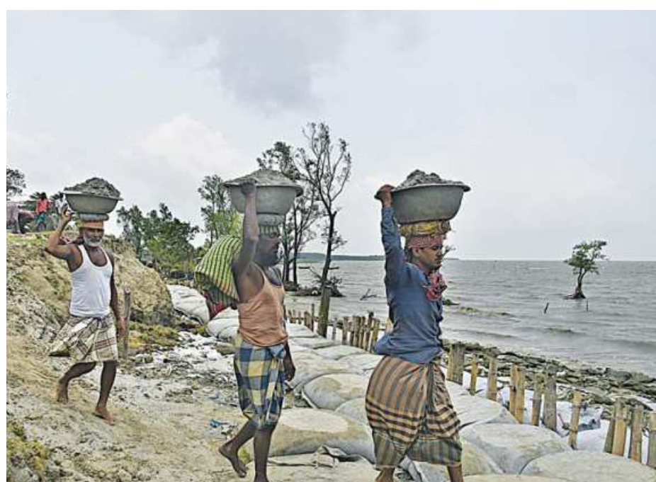
Villagers in Barguna's Patharghata upazila carrying baskets filled with sand to be put in geo bags in order to repair an embankment along the Baleswar river that was breached by tidal surges during Cyclone Yaas. The photo was taken on Monday.
