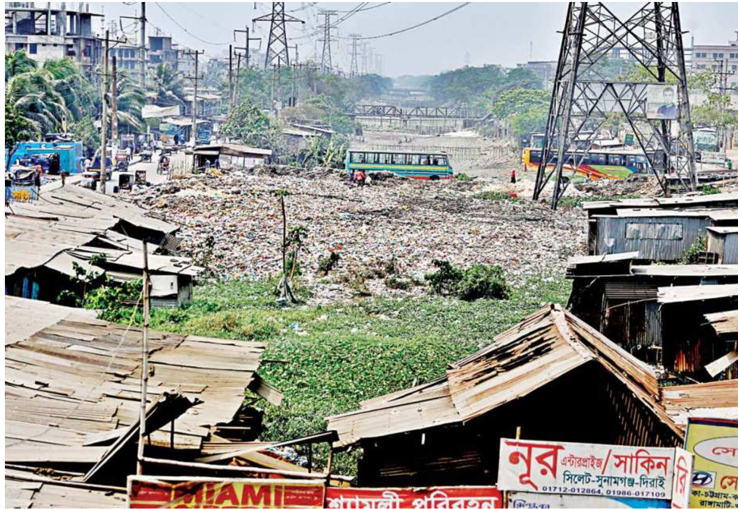
The DND canal in Narayanganj's Shiddhirganj has been turned into a landfill, blocking the canal entirely. Local influential people have built shops and other structures on the almost 1.5km long stretch. The photo was taken recently.
