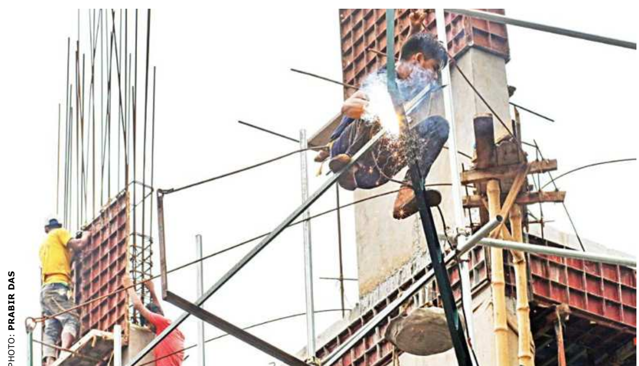
A worker barely balances himself on two thin rods, welding a safety shed on the fifth level of an under-construction building to prevent any debris from falling on passers-by. But there is no safety equipment, or even a helmet for the worker himself as he risks his life at the site. This photo was taken from Kazi Nazrul Islam Avenue in Dhaka recently.
