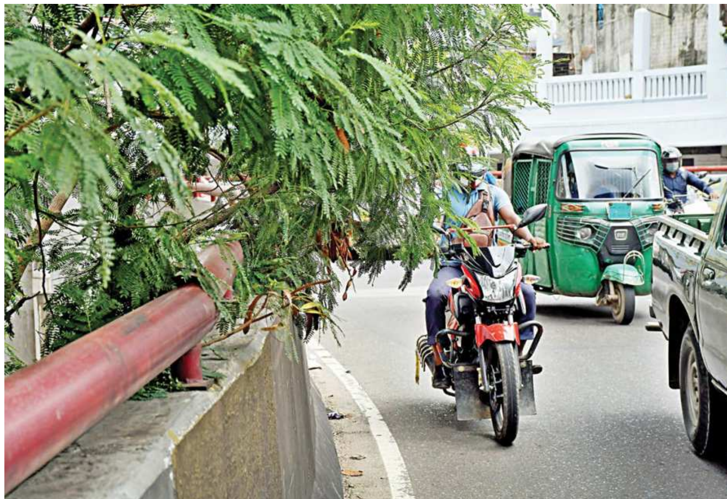
A tree dangerously leans on to the Mouchak-Malibagh flyover in the capital. Vehicles could hit it and get damaged. Motorists making the turn are also blind to what lies ahead. A simple trimming job could make the turn safer. The photo was taken yesterday.
