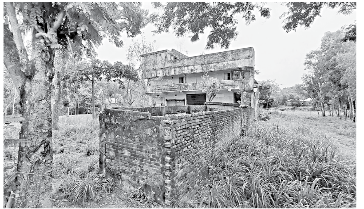
An abandoned cinema hall in Tangail's Delduar upazila.
