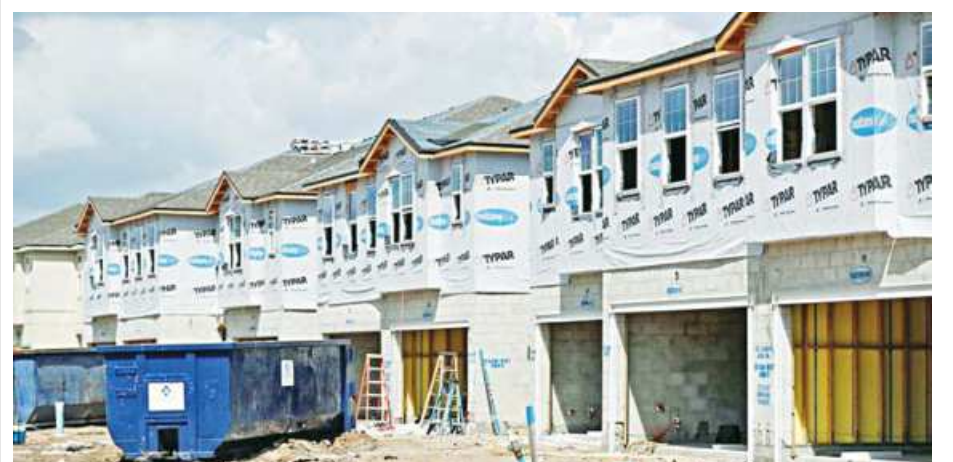
New townhomes are seen under construction while building material supplies are in high demand in Tampa, Florida.
