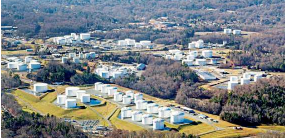
Holding tanks are seen at Colonial Pipeline's Charlotte Tank Farm in Charlotte, North Carolina, US.
