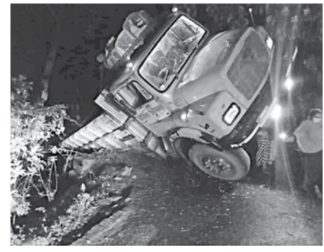
The worn-out bridge on a canal in Tangail's Nagarpur upazila collapses when a sand-laden truck was crossing it on Friday night.
