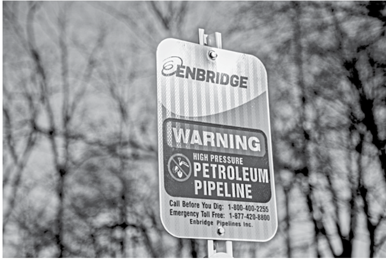
A signpost marks the presence of Enbridge's Line 5 pipeline, which Michigan Governor Gretchen Whitmer ordered shutdown in May 2021, in Ontario, Canada.
