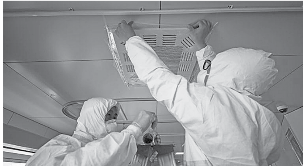
Hospital employees in Wuhan, China seal an airvent to prevent possible airborne transmission of the new coronavirus.
