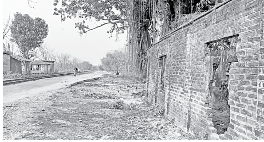
A site near the Teesta Railway Bridge in Lalmonirhat Sadar upazila. PHOTO: STAR
