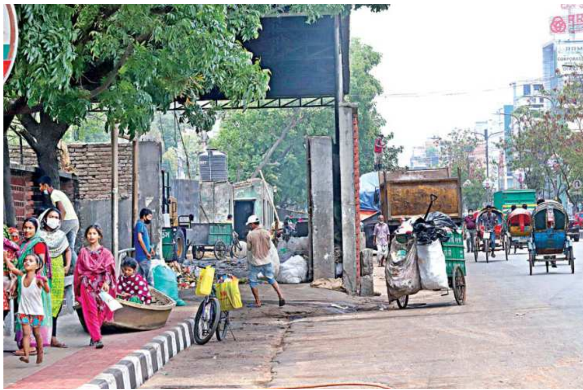
A part of the footpath on Pragati Sarani is taken up by one of DNCC's secondary waste transfer stations, built encroaching the space. To solve one problem, the corporation created another one, as pedestrians must now jaywalk around the structure while dodging traffic. While officials point to space constraints for constructing the station this way, urban planners think an alternative would have been possible through proper planning. The photo was taken yesterday.
