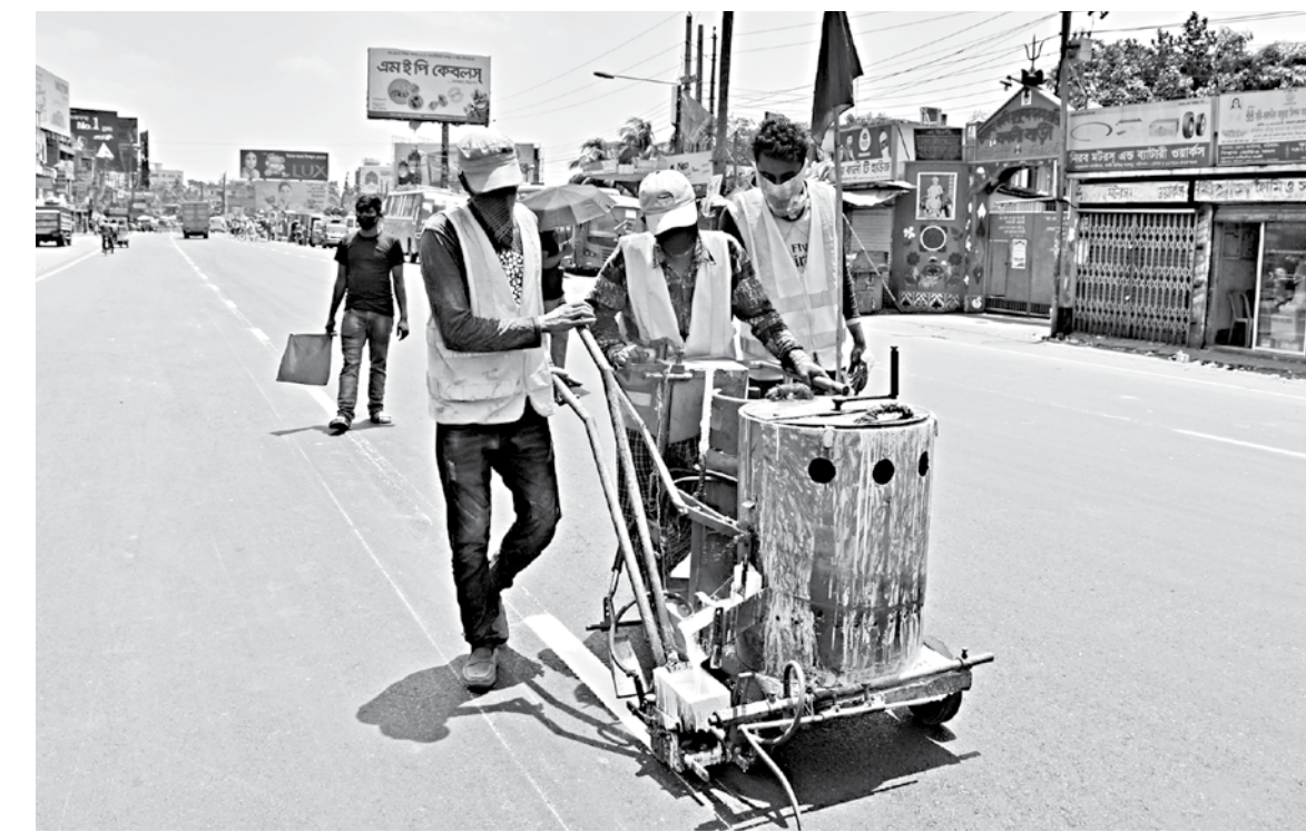
Workers mark the lanes on Barishal-Dhaka highway using their machine, and with the lockdown still in effect, little to no vehicular movement can be seen near them. Such work is perhaps easier to do in these unusual situations. This photo was taken yesterday from Barishal city's Kashipur area.
