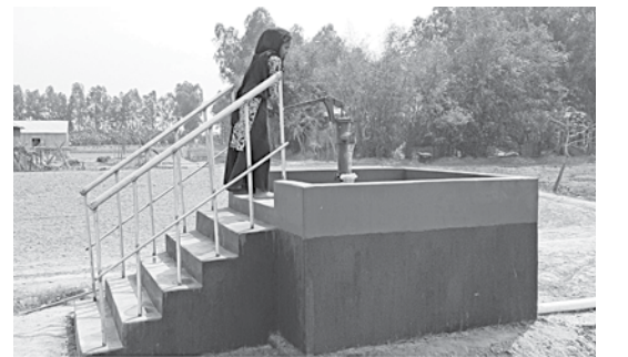
The ultra-poor families of four villages in Tangail Sadar upazila have been provided with tube wells on elevated basement under the IFRC project.
