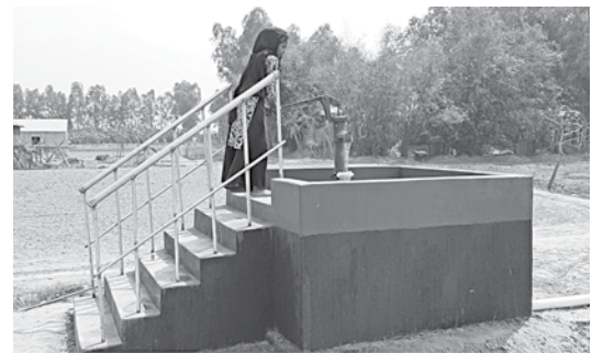
The ultra-poor families of four villages in Tangail Sadar upazila have been provided with tube wells on elevated basement under the IFRC project.
