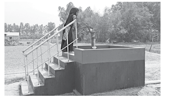
The ultra-poor families of four villages in Tangail Sadar upazila have been provided with tube wells on elevated basement under the IFRC project.
