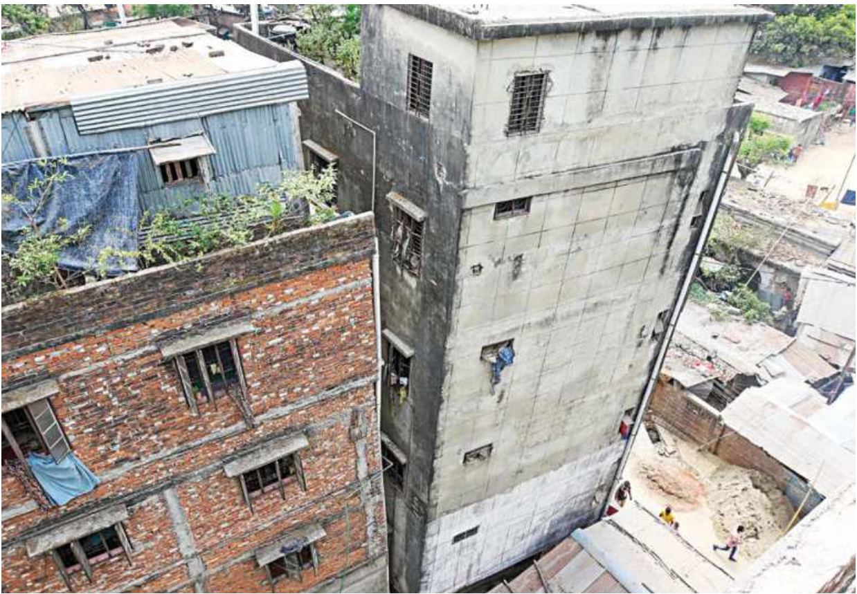
A five-storey building in port city's Enayetbazar area tilted around 9:30pm on Saturday night while piling was undergoing on the ground floor.
