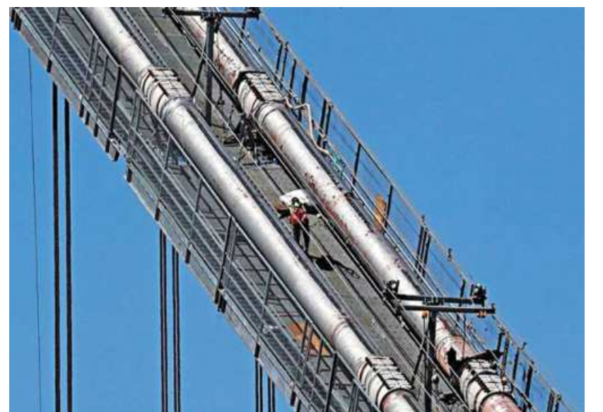
A construction worker scales the northeast cables of the George Washington Bridge, which is undergoing a multi-year reconstruction in New York City.
