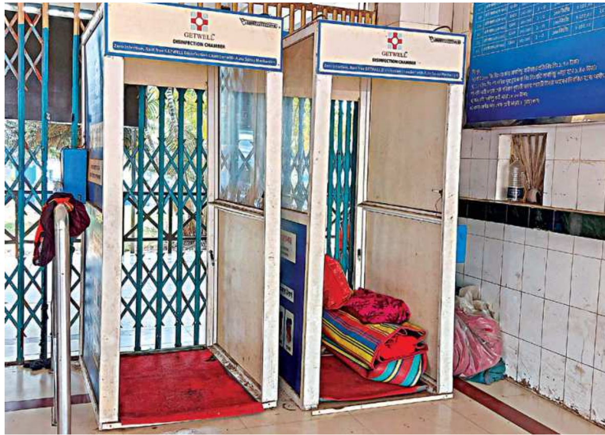
Disinfection booths in front of the ticket counters at Barishal River Port are being used for storage about a year into their installation. With proper maintenance, these booths would be useful again this year, but a lack of foresight and care has rendered them useless.
