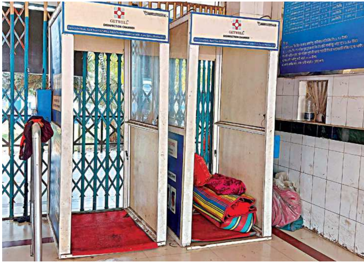
Disinfection booths in front of the ticket counters at Barishal River Port are being used for storage about a year into their installation. With proper maintenance, these booths would be useful again this year, but a lack of foresight and care has rendered them useless.
