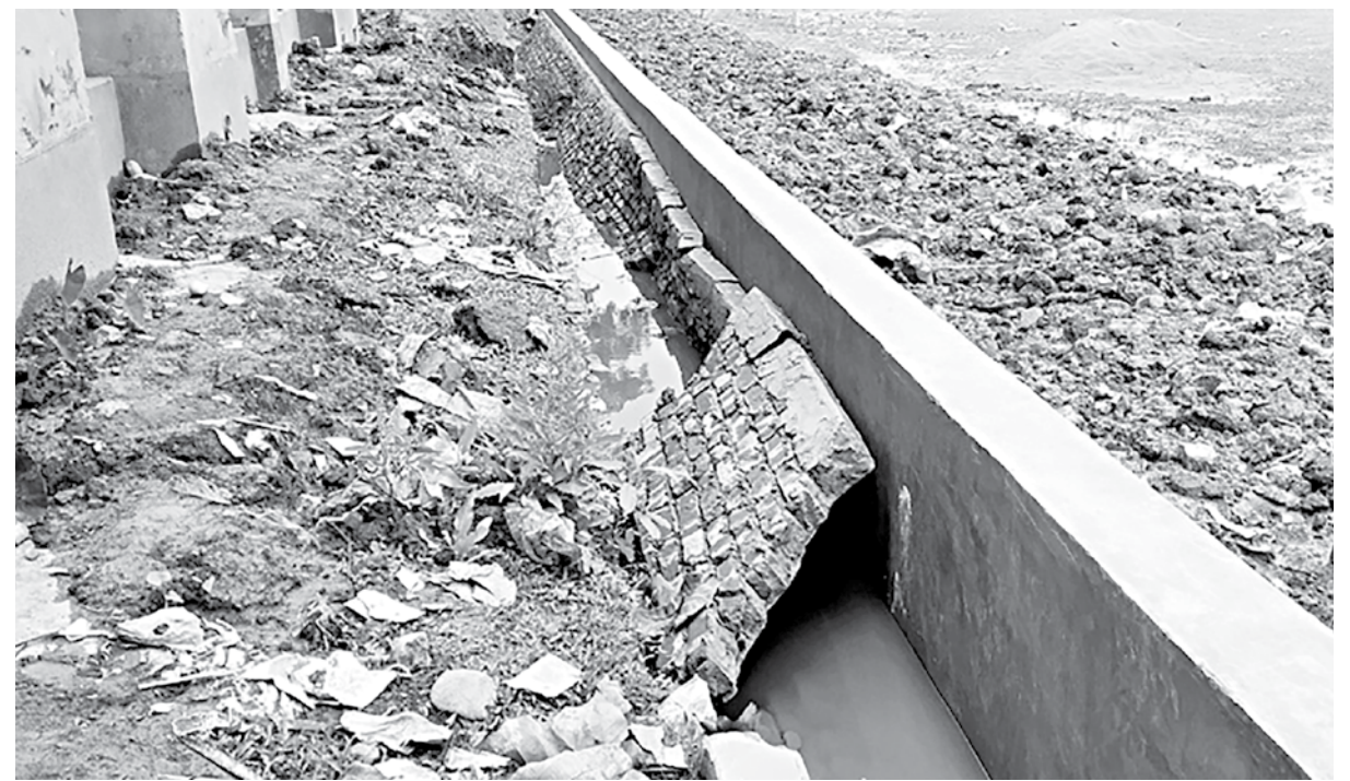
A wall of this newly built drain in Moulvibazar's Kamalganj upazila collapses on Tuesday only after 15 days of its construction. Moulvibazar district council constructed the drain, along the boundary wall of Kamalganj Government Model High School, spending Tk 2 lakh.
