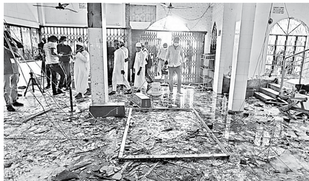
The ground floor of the mosque in Narayanganj's Talla area littered with warped blades of ceiling fans, charred remains of human flesh and prayer rugs, shards of glass and debris.
