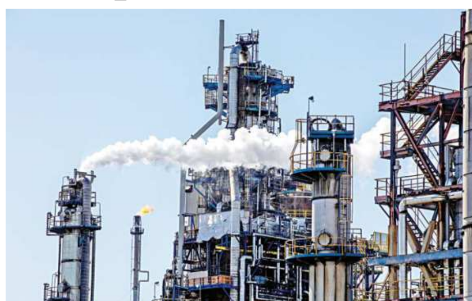
General view of the Imperial Oil refinery, located near Enbridge's Line 5 pipeline, in Sarnia, Ontario, Canada.
