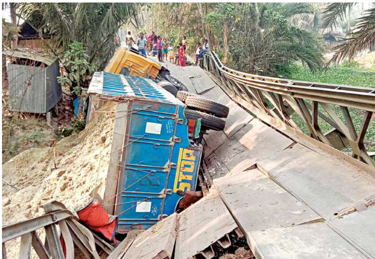
A sand-laden truck causes a Bailey bridge on the Mara Chitra river in Mollahat upazila of Bagerhat to collapse early yesterday. Bagerhat Roads and Highways Department executive engineer said there were 10 such bridges on that stretch of road and none of them could withstand so much load.
