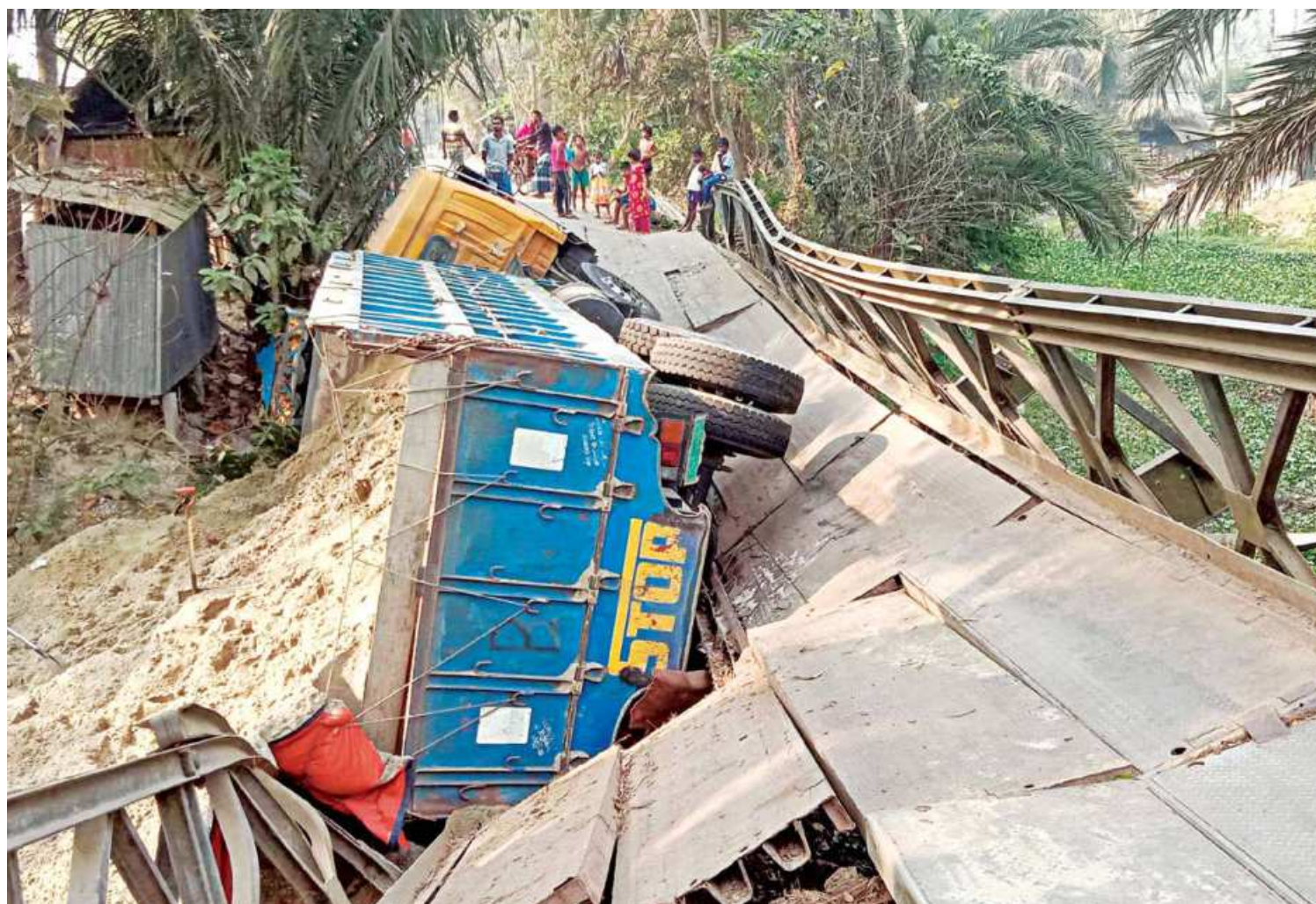
A heavily loaded sand laden truck causes a Bailey bridge on the Mara Chitra River in Mollahat upazila of Bagerhat to collapse early yesterday morning. Bagerhat Roads and Highways Department executive engineer said there were 10 such bridges on that stretch of road and none of them could withstand so much load.
