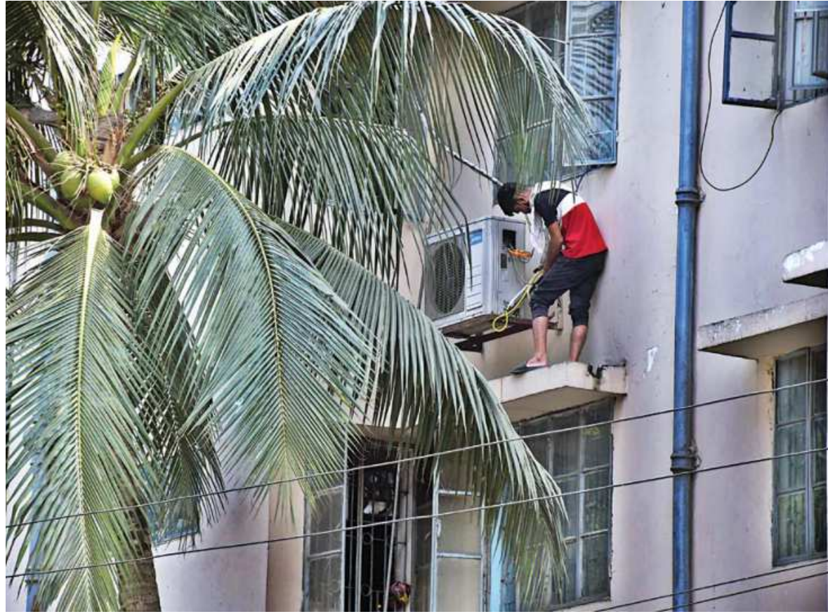
An air-conditioner mechanic stands on a narrow window ledge to fix the appliance, with no safety harness. As summer is in full gear, such mechanics can be seen in precarious positions in the coming days, neglecting safety equipment. This photo was taken yesterday from Dhaka University area.
