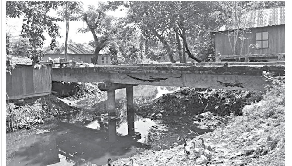
While mindless dumping of garbage in the Ichhamati river has constricted its flow in Pabna town, inconsiderate and short-sighted development -- such as this low-height bridge with its columns erected in the middle of the waterway -- by the authorities and the townspeople has made it impossible to use it as an affordable medium of transport.
