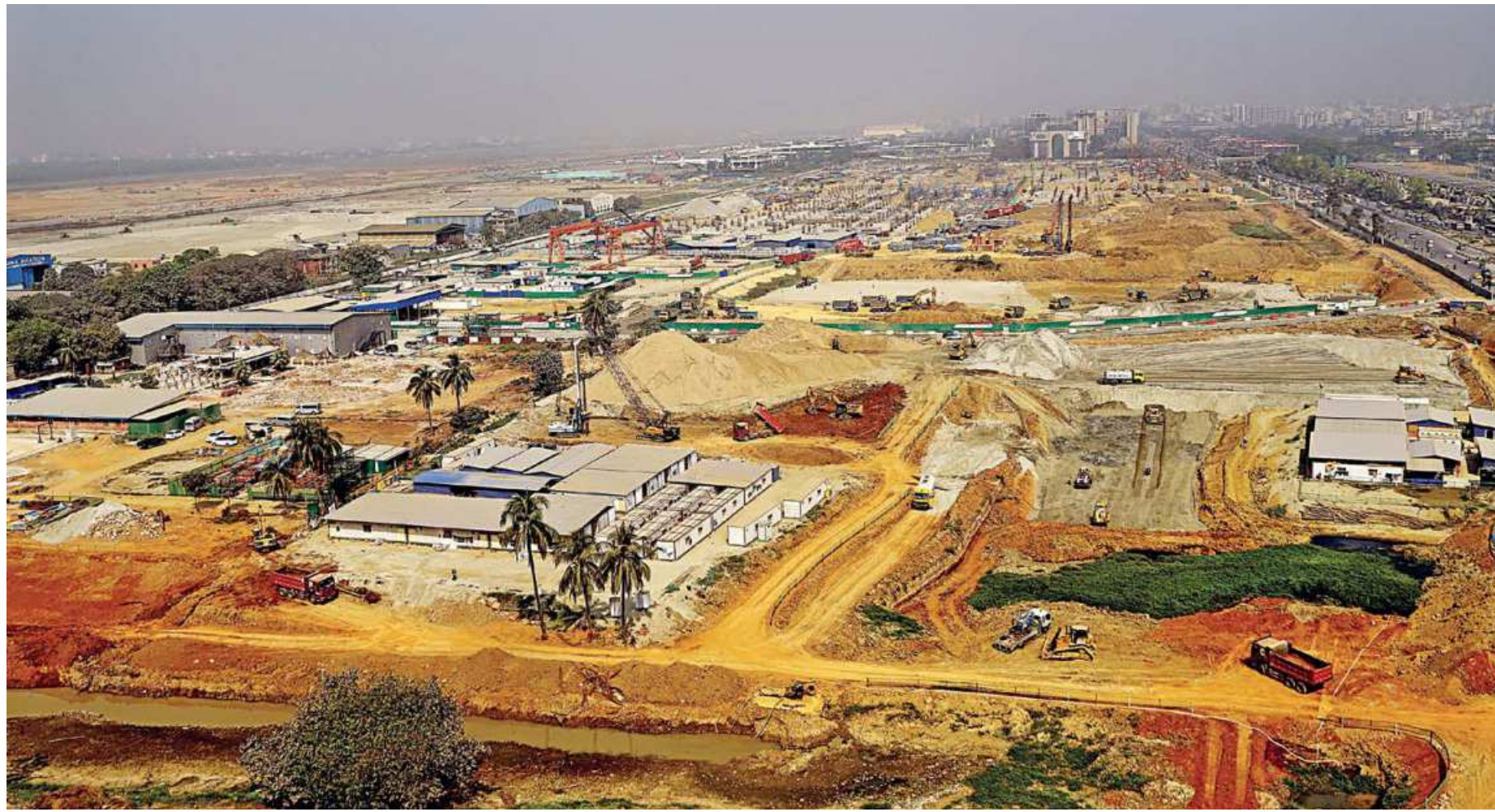
The under-construction third terminal of Hazrat Shahjalal International Airport. The Tk 21,399 crore project is funded by Jica and the Bangladesh government. Mitsubishi and Fujita of Japan and Samsung of Korea are expected to complete the work by June, 2023. The photo was taken a couple of days ago.
