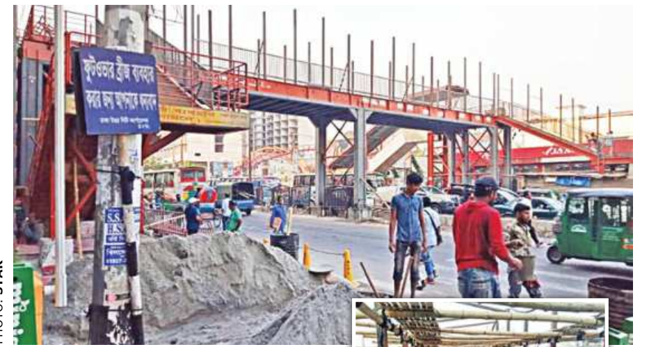
A sign saying "Thank you for using the footbridge" stands in irony on Pragati Sarani in the capital, as work continues on the structure. Inset, workers were recently seen replacing the railings of the bridge.
