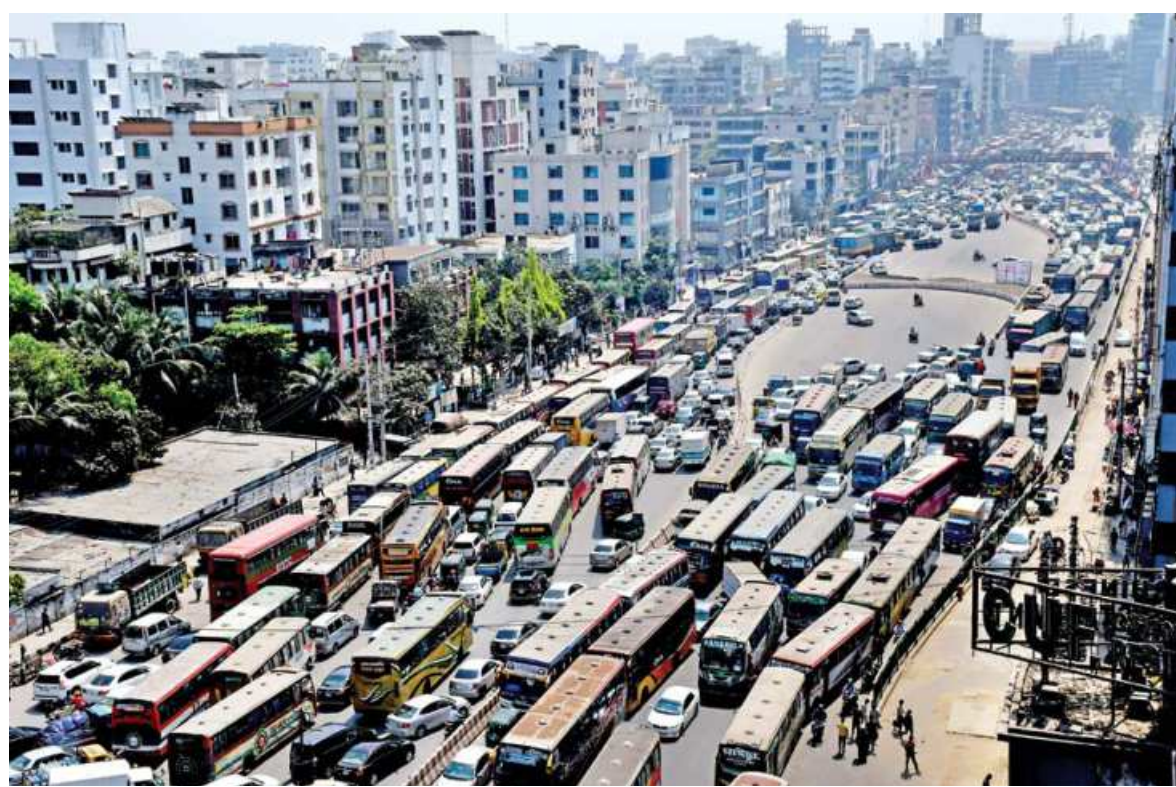
A view of the Airport Road in the capital's Uttara shows traffic at a standstill after portion of a launching girder of the Bus Rapid Transit project collapsed near the Hazrat Shahjalal International Airport. The photo was taken yesterday around 12:30pm.
