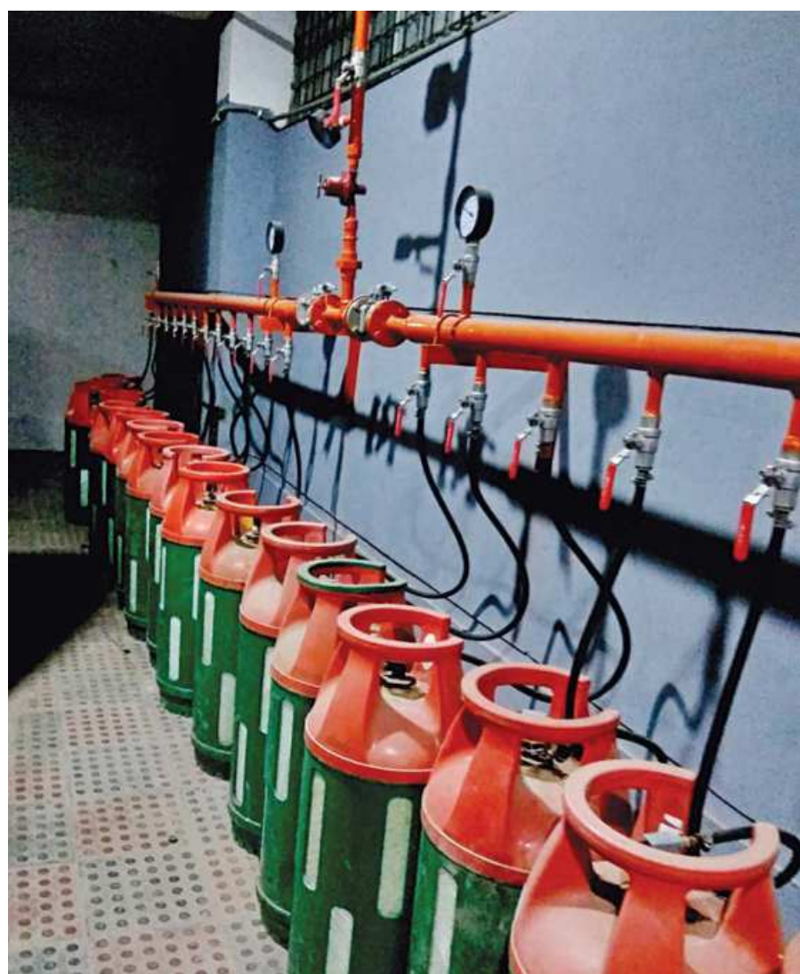
Gas cylinders lined up on the ground floor of a multi-storey apartment building in Ulon area of Rampura in the capital. The cylinders are kept there and connected to the kitchens upstairs using pipes as the apartment residents fear that the cylinders might explode. The photo was taken yesterday.
