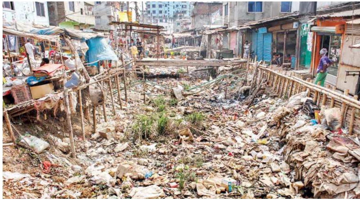
This canal in Jatrabari's Kajla has been in this shambolic state for a long time. Even though DSCC has launched a cleaning and eviction drive here, the sheer size of the canal and the amount of waste dumped in it is delaying completion of the works. This photo was taken on March 1.
