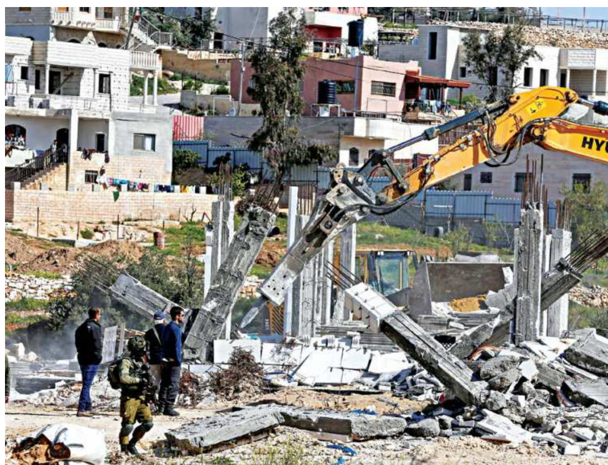
A machinery guarded by Israeli forces demolishes an under-construction Palestinian building, in Bani Naim near Hebron in the Israeli-occupied West Bank yesterday.
