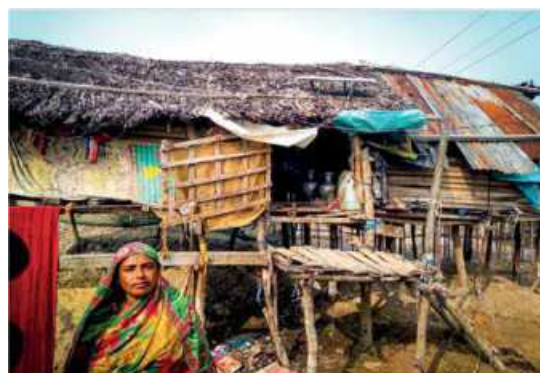
"Our village gets inundated every day during the tidal surges, water breaks in through the damaged part of the embankment" - Rahima Khatun (43), Day laborer
