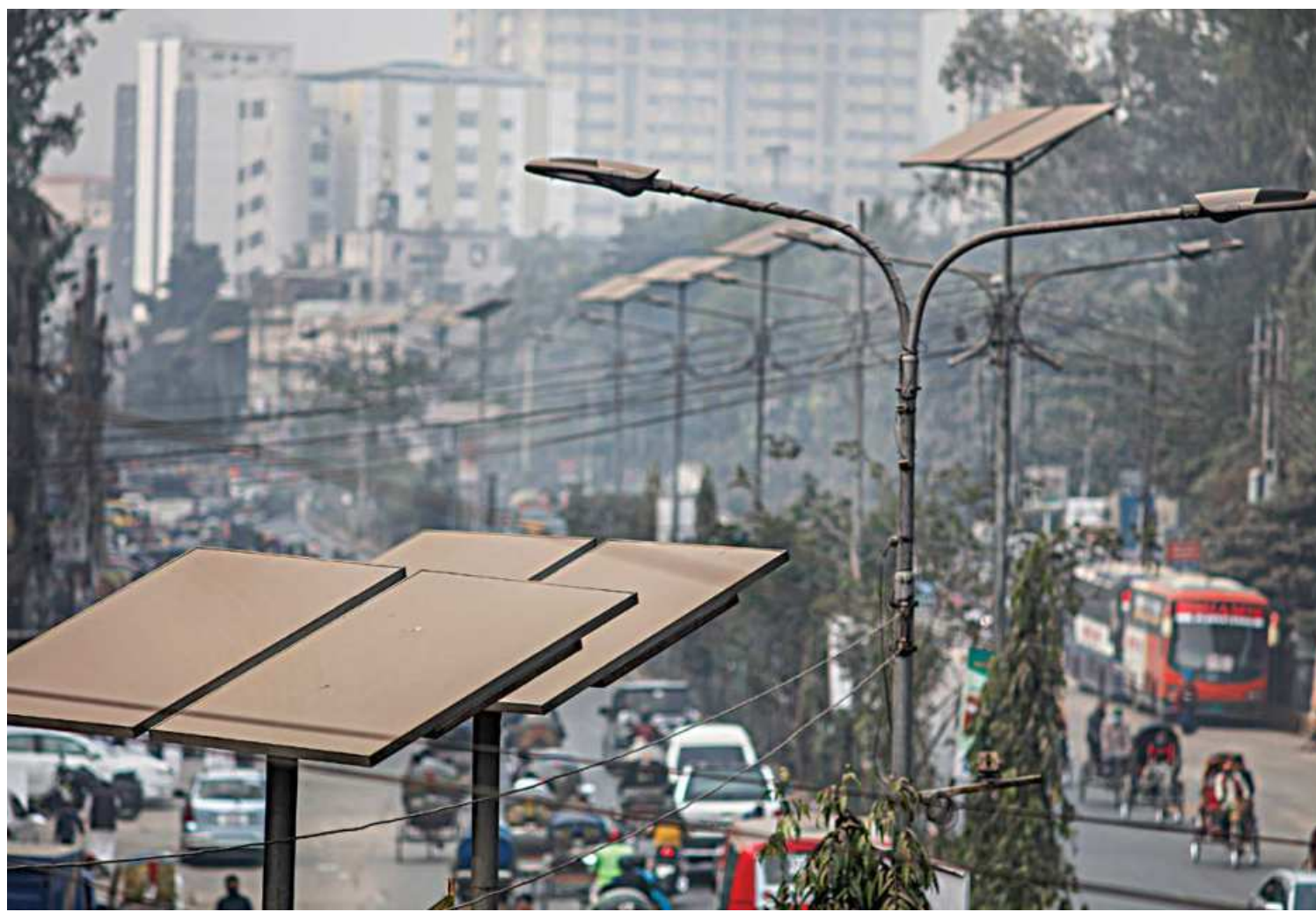
A thick layer of dust on the solar panels that recharge the street lights in Fakirpool area of the capital. If the panels are not cleaned properly at regular intervals, it renders them unable to generate adequate amount of power from the sun.
