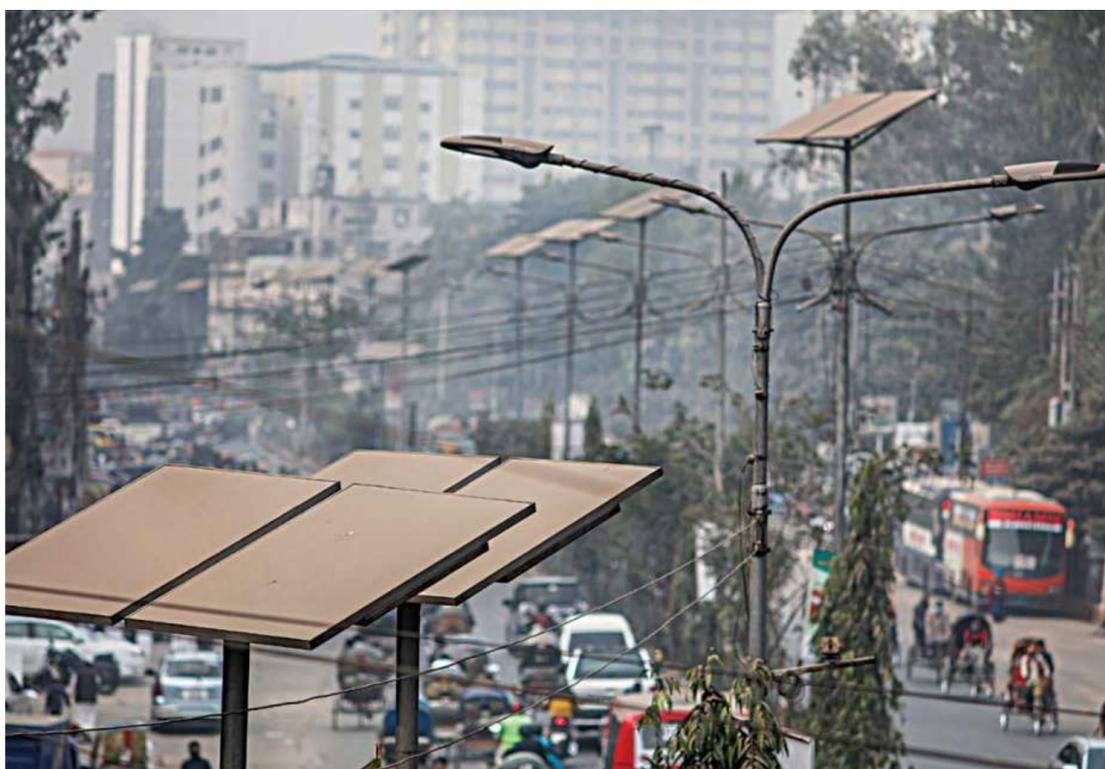
A thick layer of dust on the solar panels that recharge the street lights in Fakirpool area of the capital. If the panels are not cleaned properly at regular intervals, it renders them unable to generate adequate power from the sun.
