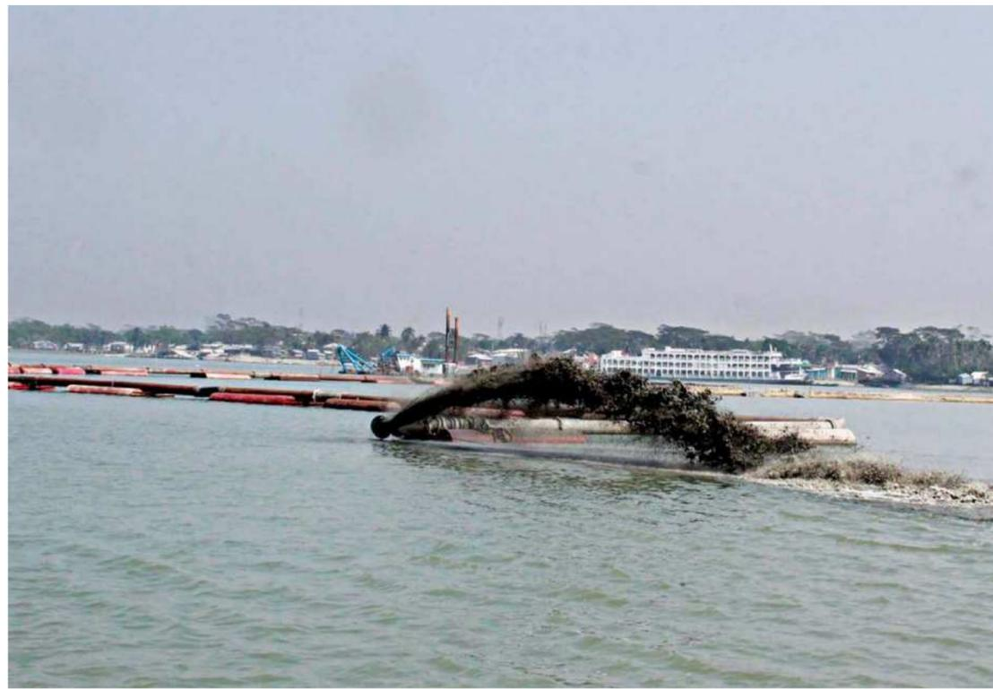
Discharge from a dredger is being dumped straight into the Payra river near Amtali Ferry Terminal in Barguna making the dredging efforts futile as the silt will eventually clog up another part of the river key for water transport. The photo was taken recently.
