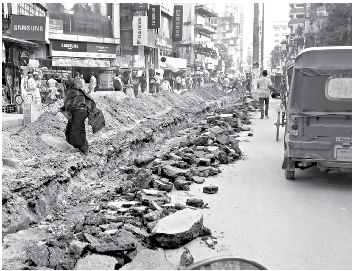
The main road of Sylhet city's Amborkhana area is dug almost down the middle for repair work on the area's water supply. This is taking its toll on pedestrians, vehicular movement, as well as on the busy area's entrepreneurs. Locals say their day-to-day activities would be far less disrupted if the development work was carried out from 8pm-6am instead of daytime. This photo was taken on Sunday.
