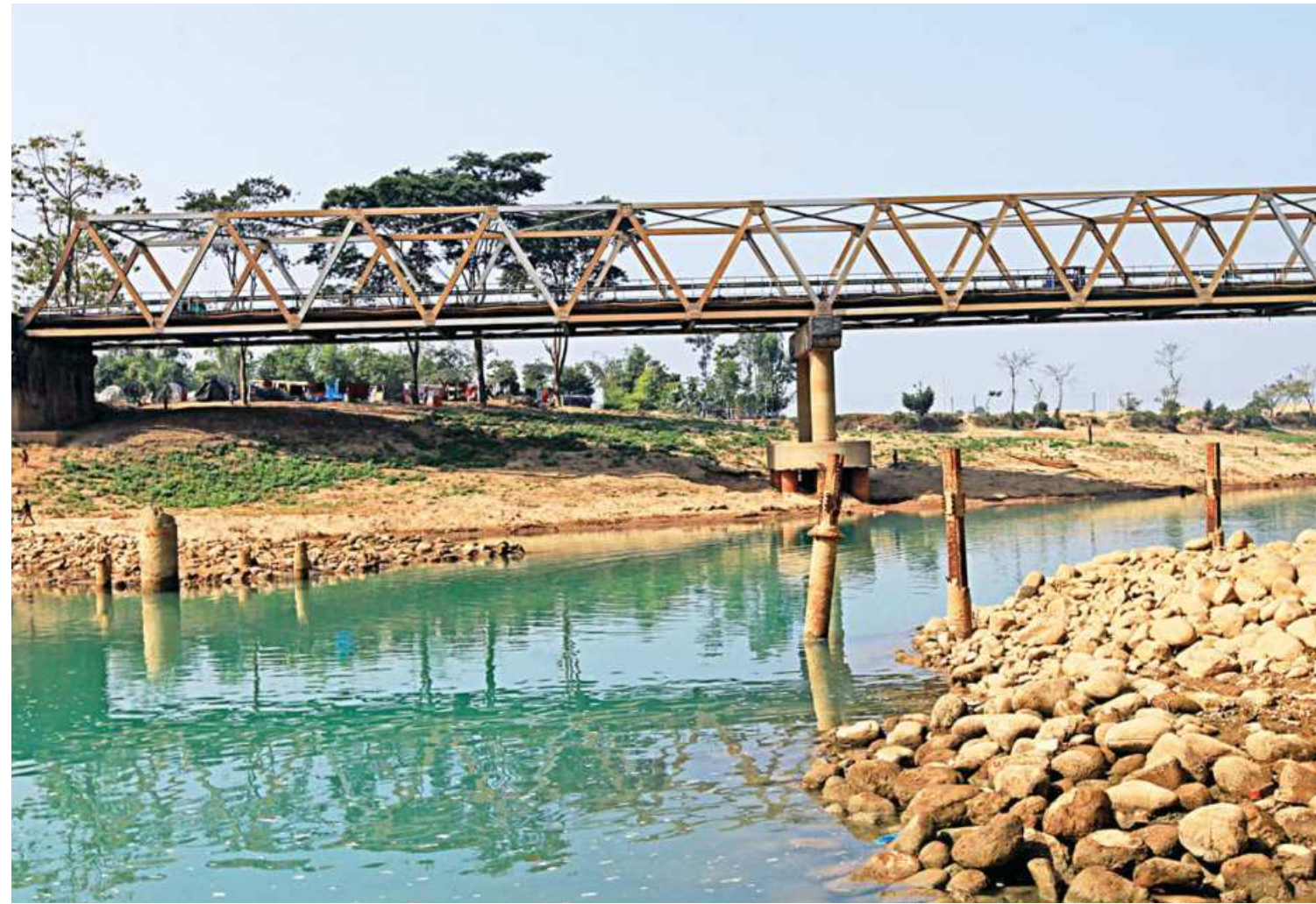
The authorities did not remove the remains of a decommissioned bridge on the Sylhet-Shillong highway even though a new bridge was built around 20 years ago. The pilings have helped reduce the navigability of the river which has shrunk significantly over the years.
