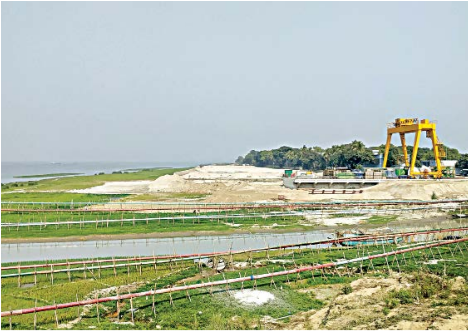
Sand from the Meghna being pumped to the shore via large pipes to fill up the bank to construct a new Ashuganj Power Plant unit in Brahmanbaria. The photo was taken recently.
