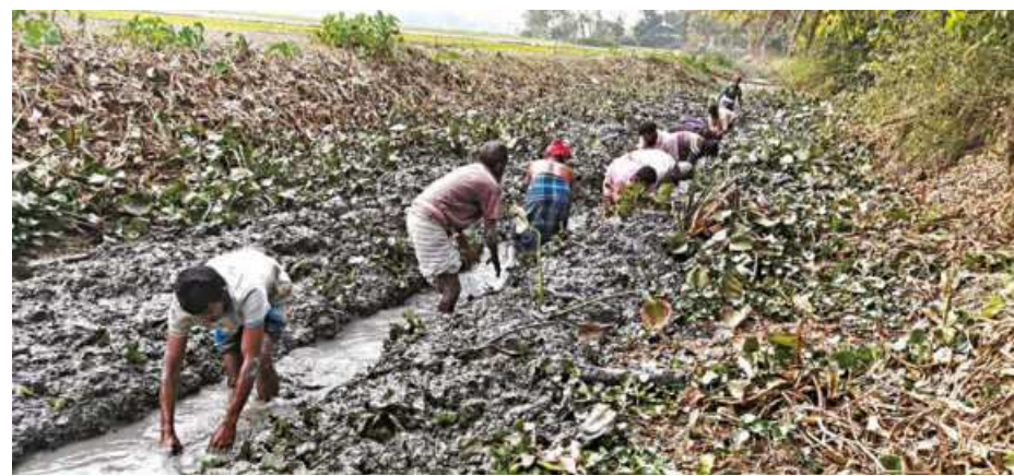
Local volunteers prepare a canal for re-excavation. The two-kilometre long Jauta-Naumala-Boga canal, in Patuakhali's Baulal upazila, has been dormant for around two decades.
