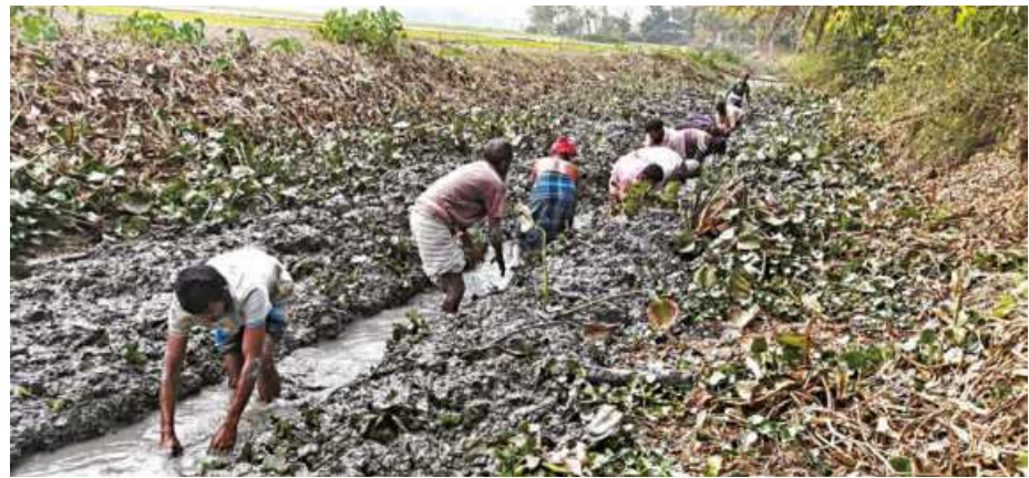
Local volunteers prepare a canal for re-excavation. The two-kilometre long Jauta-Naumala-Boga canal, in Patuakhali's Baulal upazila, has been dormant for around two decades. PHOTO: SOHRAB HOSSAIN
