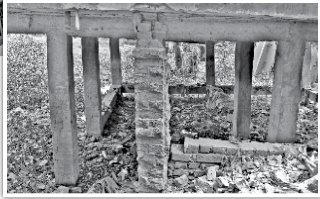
Near the Charail playground in the capital's Keraniganj where a three-storey building toppled on its side on Friday, a number of other buildings stand on concrete pillars going into wetlands, one of them six-storied. Some building owners have even put additional bricks to support their building (inset). Each of these establishments, presumably erected flouting legal guidelines, is a tragedy waiting to happen. The photos were taken yesterday.
