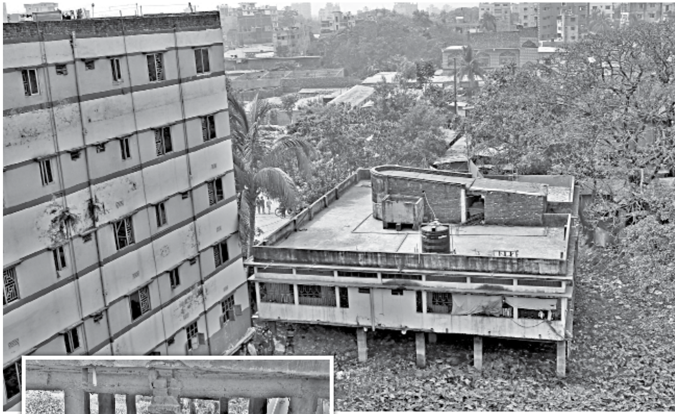
Near the Charail playground in the capital's Keraniganj where a three-storey building toppled on its side on Friday, a number of other buildings stand on concrete pillars going into wetlands, one of them six-storied. Some building owners have even put additional bricks to support their building (inset). Each of these establishments, presumably erected flouting legal guidelines, is a tragedy waiting to happen. The photos were taken yesterday.
