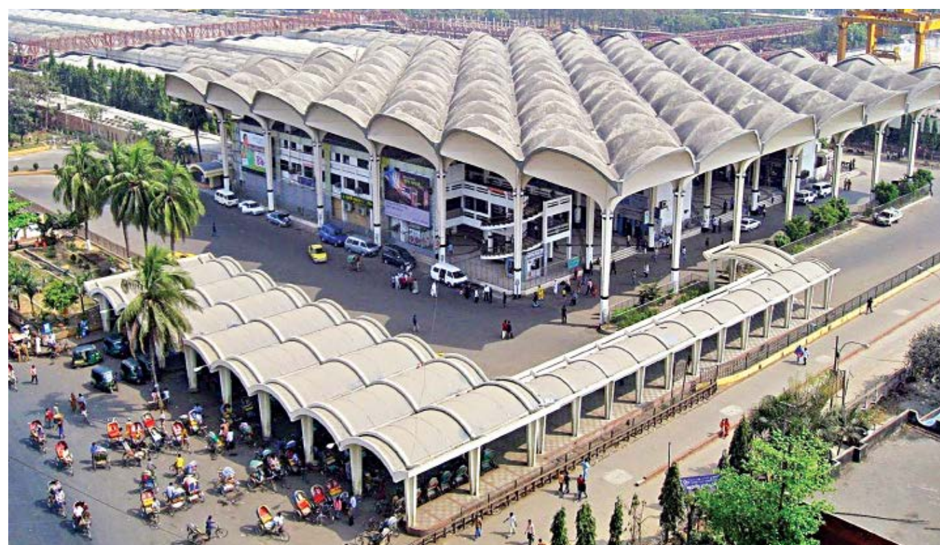
Kamalapur Railway Station.
